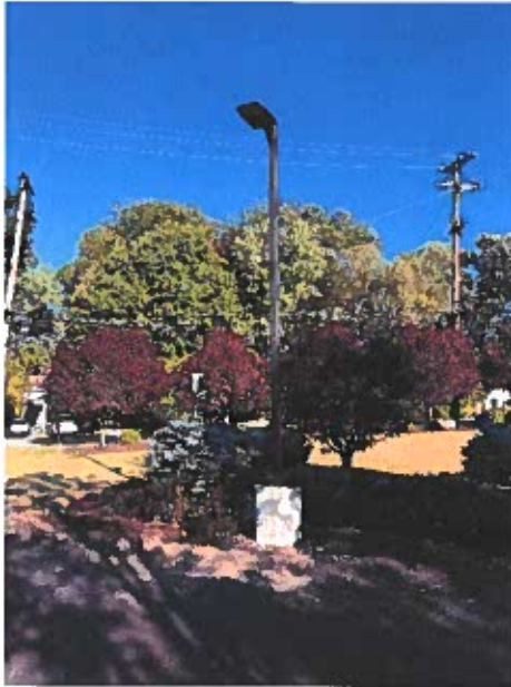
Light pole and base.
