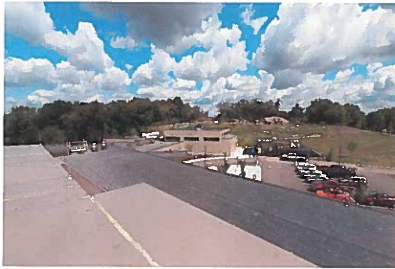
Excess dirt being removed from site.
