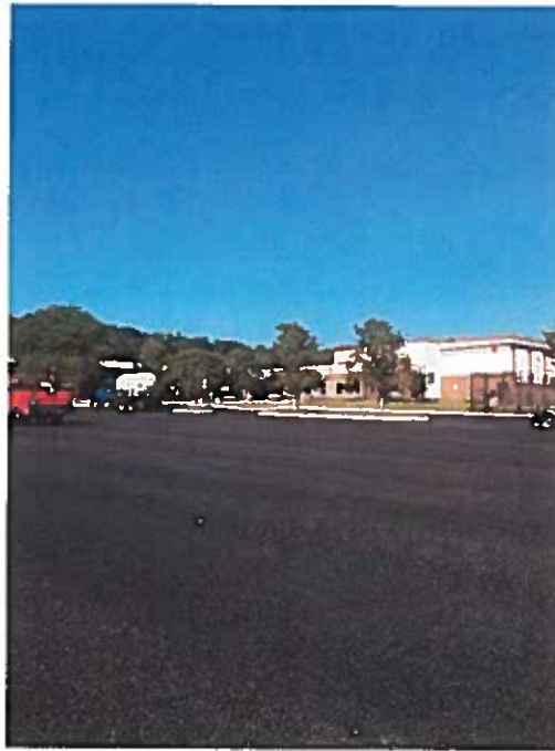
Binder completed on the large parking lot.
