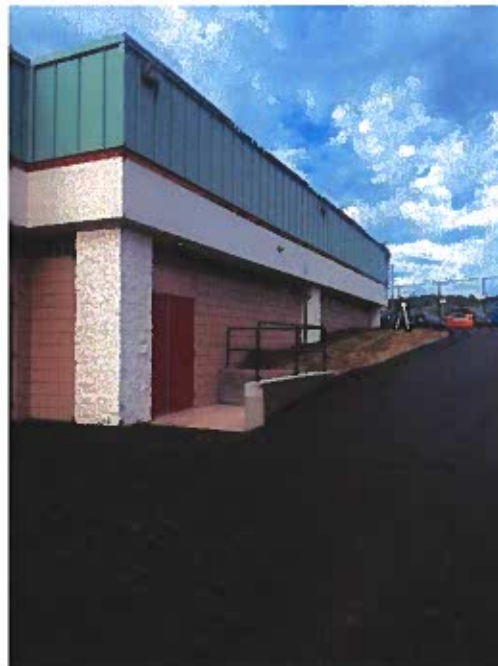
New retaining wall completed.
