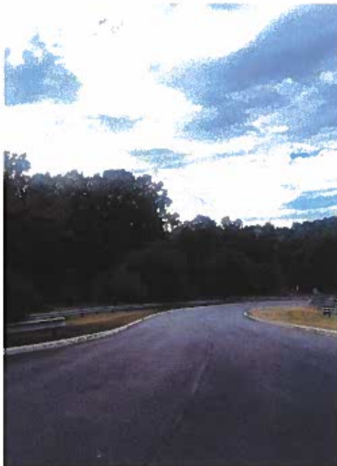
Wearing course installed on upper main entry.
